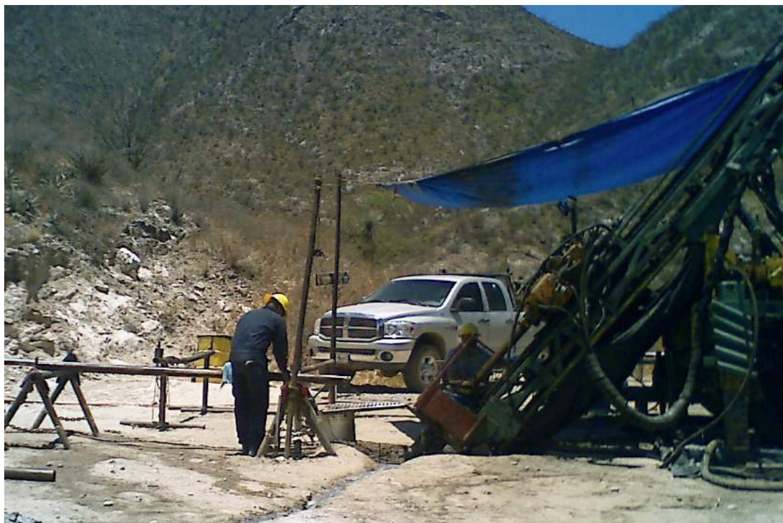
Figure 20: View of hydraulic drill from Layne de Mexico S.A. de C.V.
