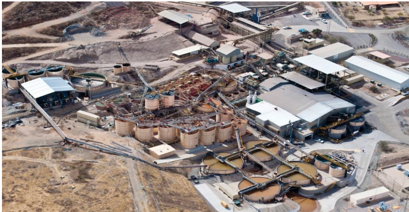
Figure 2 – View of the La Parrilla Mill Complex
